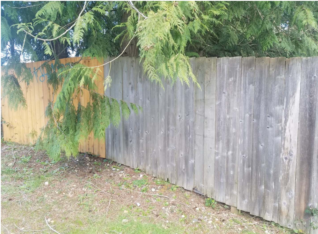
Existing fence along North Creek Drive.
