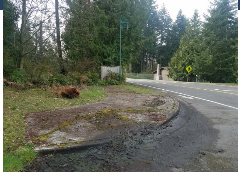
View from the access drive looking south toward the City property
